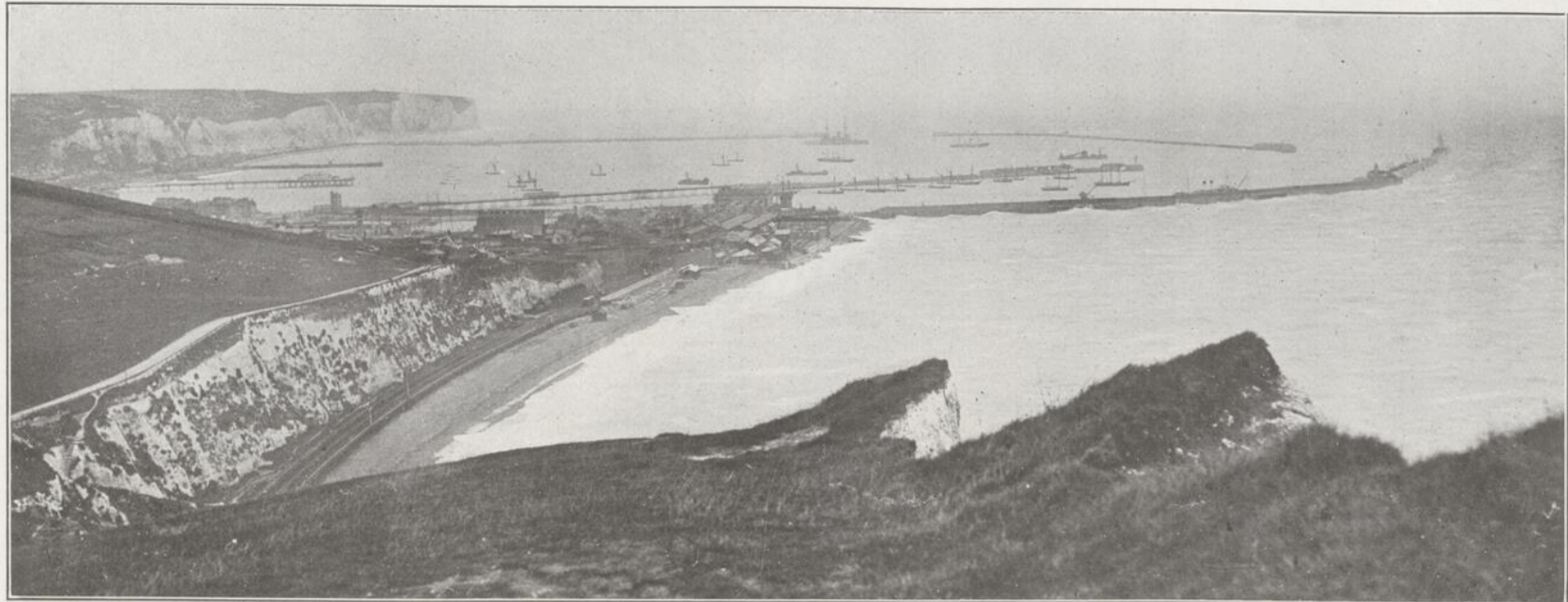
THE NEWEST NAVAL PORT IN GREAT BRITAIN—The national harbor at Dover, Eng., which was recently opened by H.R.H. the Prince of Wales. It is the result of twelve years' arduous work, and consists of a naval basin 610 acres in extent and a tiny commercial basin of 80 acres. The harbor is enclosed by the Admiralty Pier, 4,000 feet long; the "eastern" arm, 3,320 feet long; and the detached southern breakwater, 4,200 feet long. During the twelve years of work, as many as 2,000 men were employed at one time.
