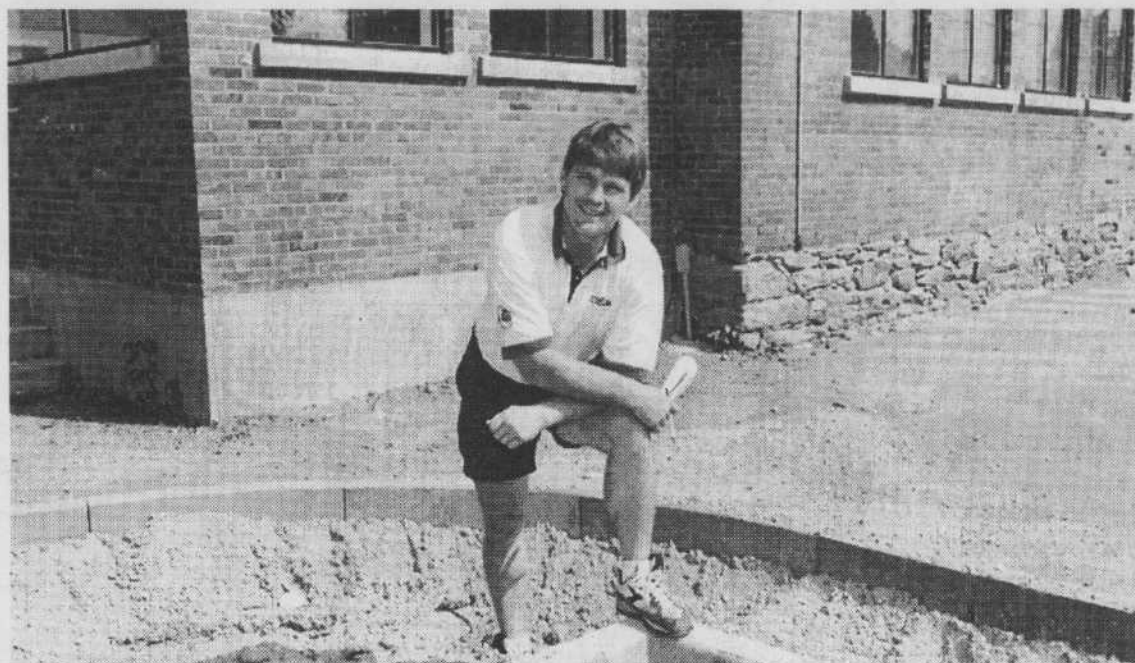
Peter MacLean installed concrete blocks to stop the flow of traffic through his Lennoxville parking lot.
