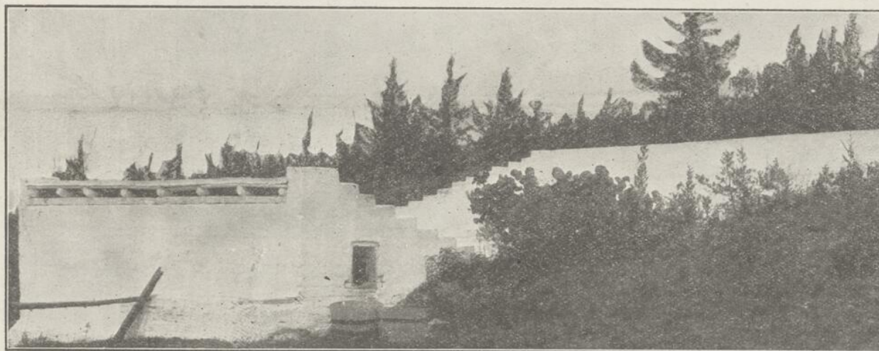
LOVELY BERMUDA, THE WINTER HOME OF MANY CANADIANS—It being impossible to secure fresh water in any other way (owing to the porosity of the rock, which causes the latter to absorb the rain-falls at once), all the water used for domestic purposes is caught from the rain-falls in reservoirs or tanks. The illustration shows one of these reservoirs, together with a "water-catch." The latter is placed on the slops of a hill, and as the rain descends, the water is caught therein.
