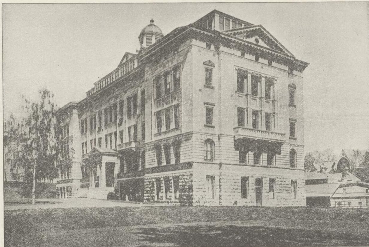
MACDONALD COLLEGE AT ST. ANNE DE BELLEVUE, NOW UNDER JURISDICTION OF MCGILL, RECALLS FORMER MAGNIFICENT GIFTS OF SIR WILLIAM MACDONALD TO THE UNIVERSITY—The Engineering Building at McGill, the first of Sir William's structural donations to McGill.
