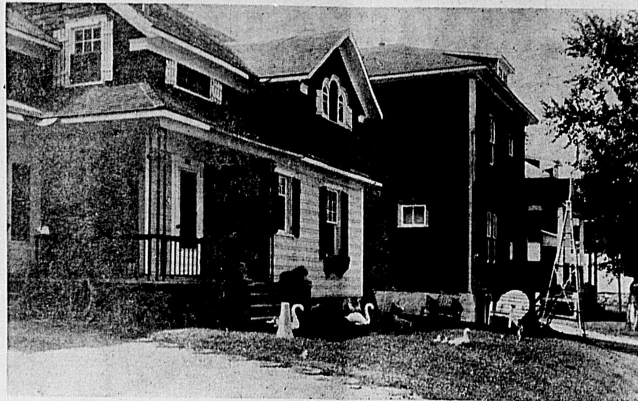
Showing the home of Mr. and Mrs. Jim Proulx, 224 Roy Street, long-time residents of Thetford Mines, and their lawn ornaments in the form of dogs, swans, ducks and ducklings, and two lions guarding the entrance.
