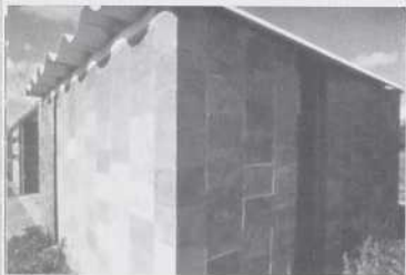
ECOL Operation, an experimental low-cost ecological demonstration house using interlocking sulphur blocks, which was put up on the Macdonald College by a group of Minimum Cost Housing Students under the direction of Alvaro Ortega, 1972.
