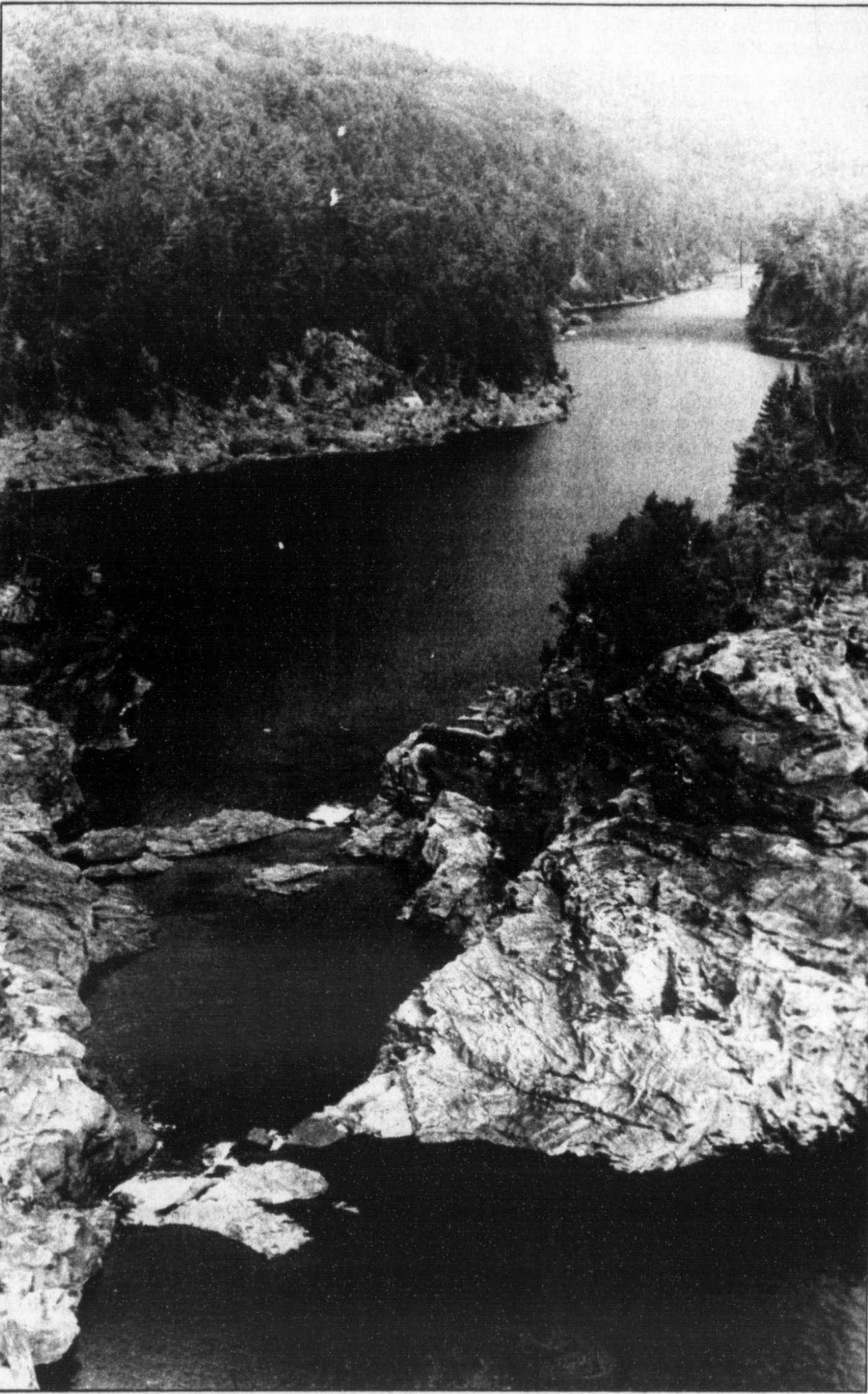
Ontario Hydro recently gave the Passe des Rapides Committee permission to build on the 400-foot flood plain area on the shore of McConnell Lake. Shown, is a view of the lake from the top of the Hydro Dam at Rapides des Joachims.
