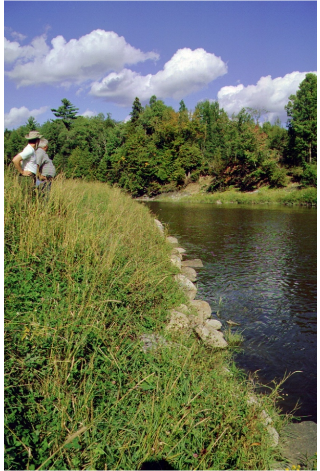
Streambank Restored with Rip-rap and Vegetative Cover
