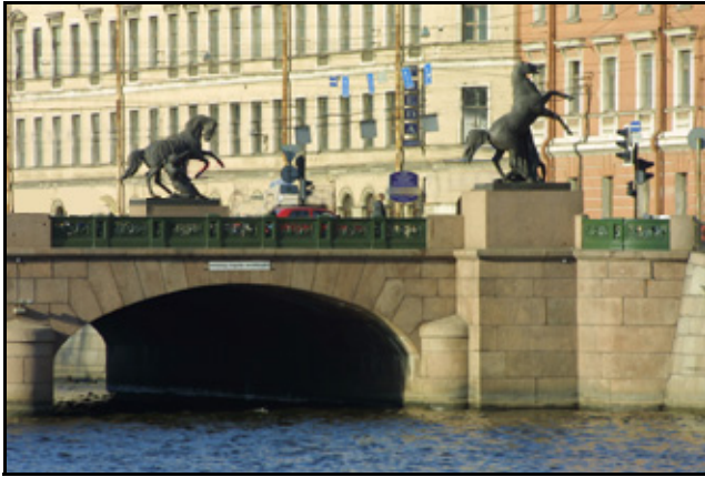
Figure 3.11: Anikhov Bridge named after the engineer who designed it.
