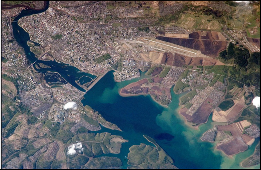
Figure 1.17: Irkutsk Hydroelectric Dam.
