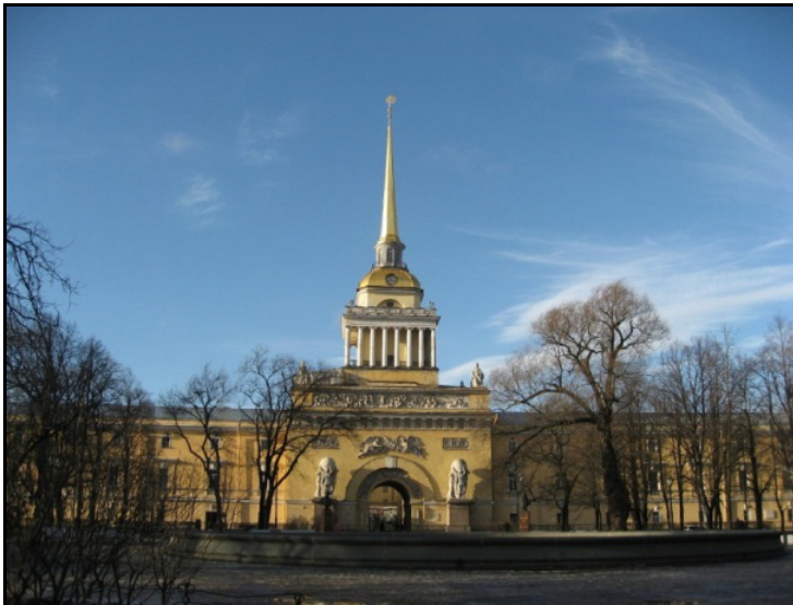
Figure 3.27: Russian Admiralty Building in Saint Petersburg.
