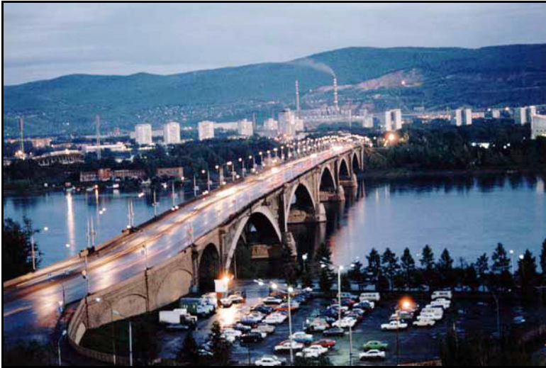
Figure 1.5: One of the three bridges across the Yenisei River.
