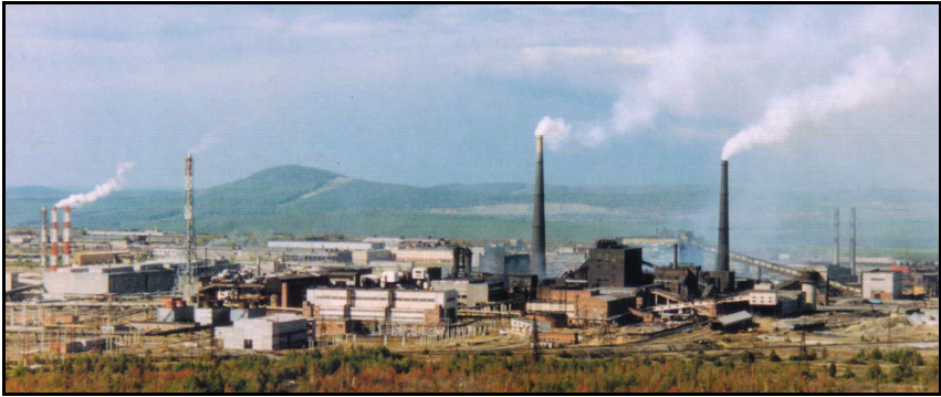
Figure 1.19: Sredneuralsky Copper Smelter at Rivda uses Vanyakov furnace, 2001.
