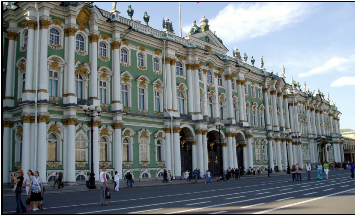
Figure 3.34: Winter Palace view from the Palace Square.
