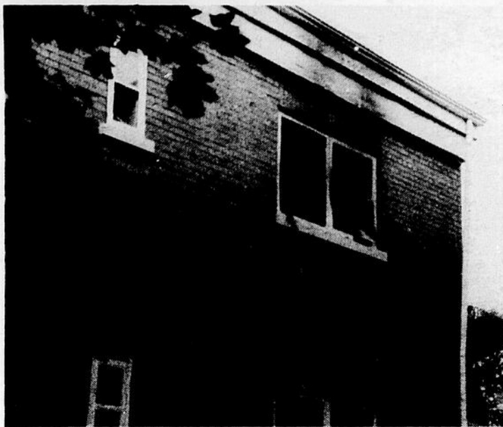
Smoke marks above the window and a dangling fire hose mark the room gutted in Monday's fire at 314 Lansdowne avenue.
