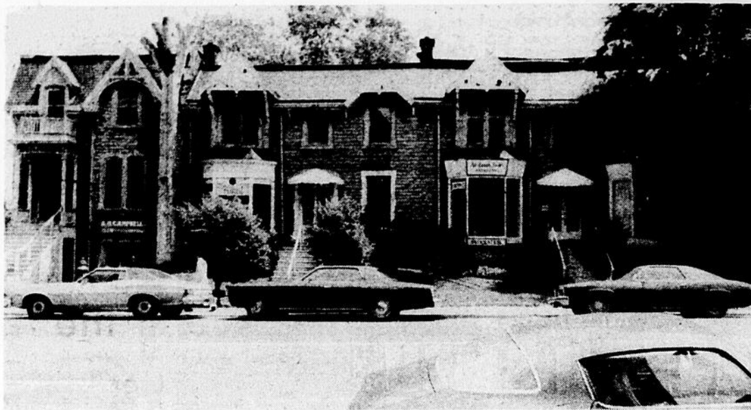
The set-back St. Catherine street buildings.
