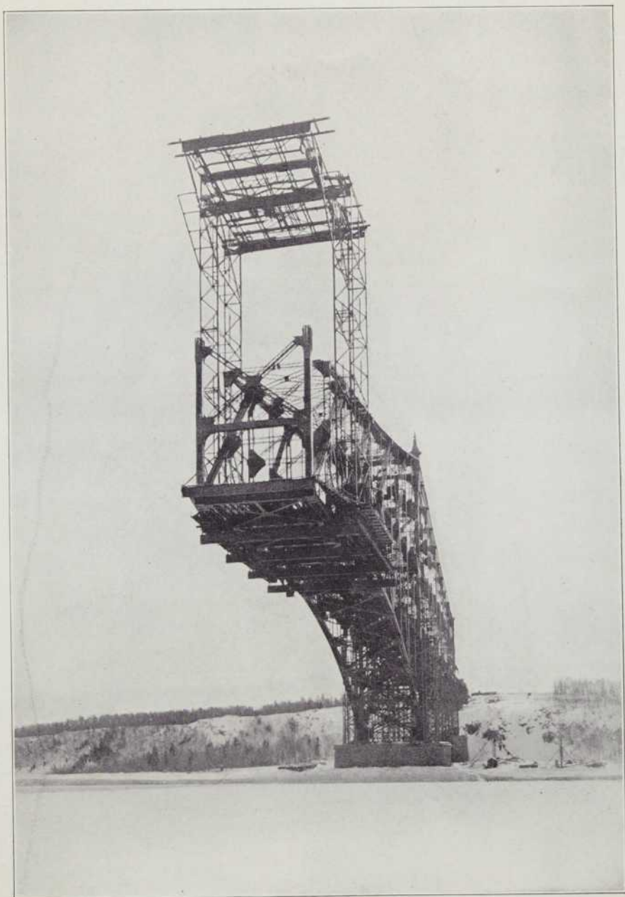
SOUTH CANTILEVER ARM FROM RIVER.
