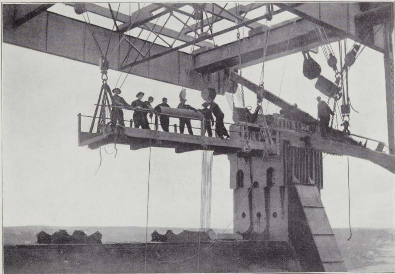
DRIVING A 12-INCH TOP CHORD PIN.
