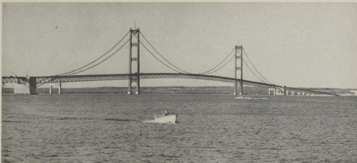
WITH THE WORLD'S SECOND LONGEST SPAN, 3,800 FEET, THE NEW STRAITS OF MACKINAC BRIDGE IS BUILT TO SHRUG OFF THE MOST POWERFUL WINDS EVER RECORDED. CONSIDERED THE SAFEST SUSPENSION BRIDGE, IT IS ALSO THE LONGEST, FROM ANCHORAGE TO ANCHORAGE.
