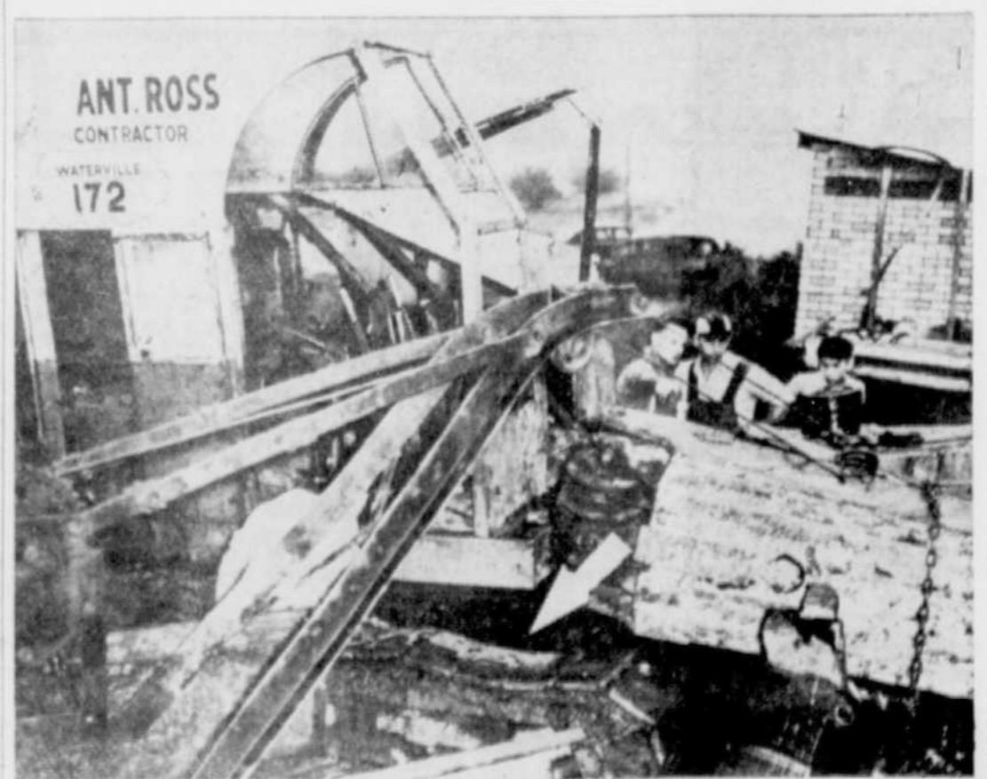
FATAL ACCIDENT — The scene of the fatal accident at North Hatley Friday evening when Antonio Ross, Waterville contractor, was crushed while repairing his steam shovel, is seen above. White arrow indicates where Ross' body fell after the boom, which weighed about 10 tons, was removed by a crane. (Record Photo by Doug Gerrish)
