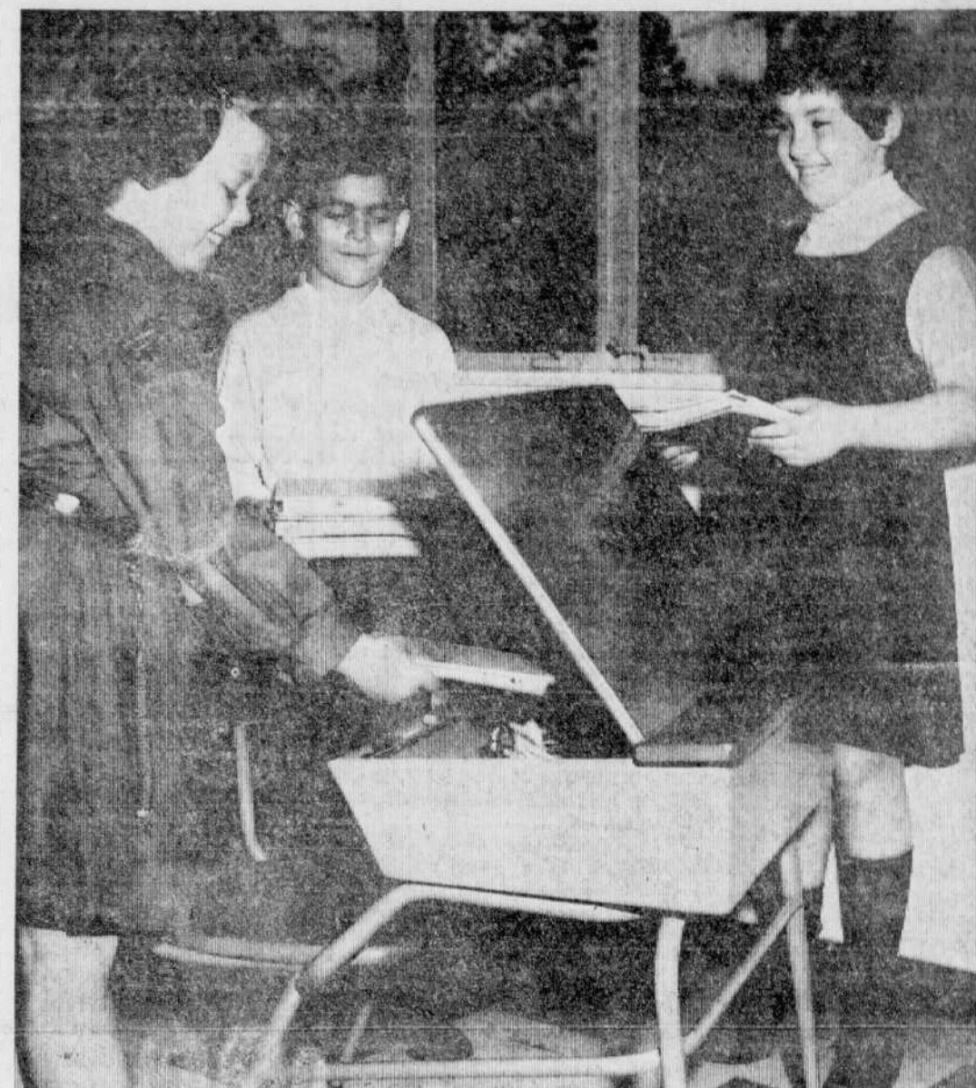
MOVING IN — Mitchell School students temporarily moved into the new addition of the school yesterday afternoon while workmen repaired the older wing of the building. Official opening of the new wing will be in October. From the left are: Carolyn Annesley, Jamie Elger and Judy Kandalaft, all grade three students. (Record Photo by Gerry Lemay)
