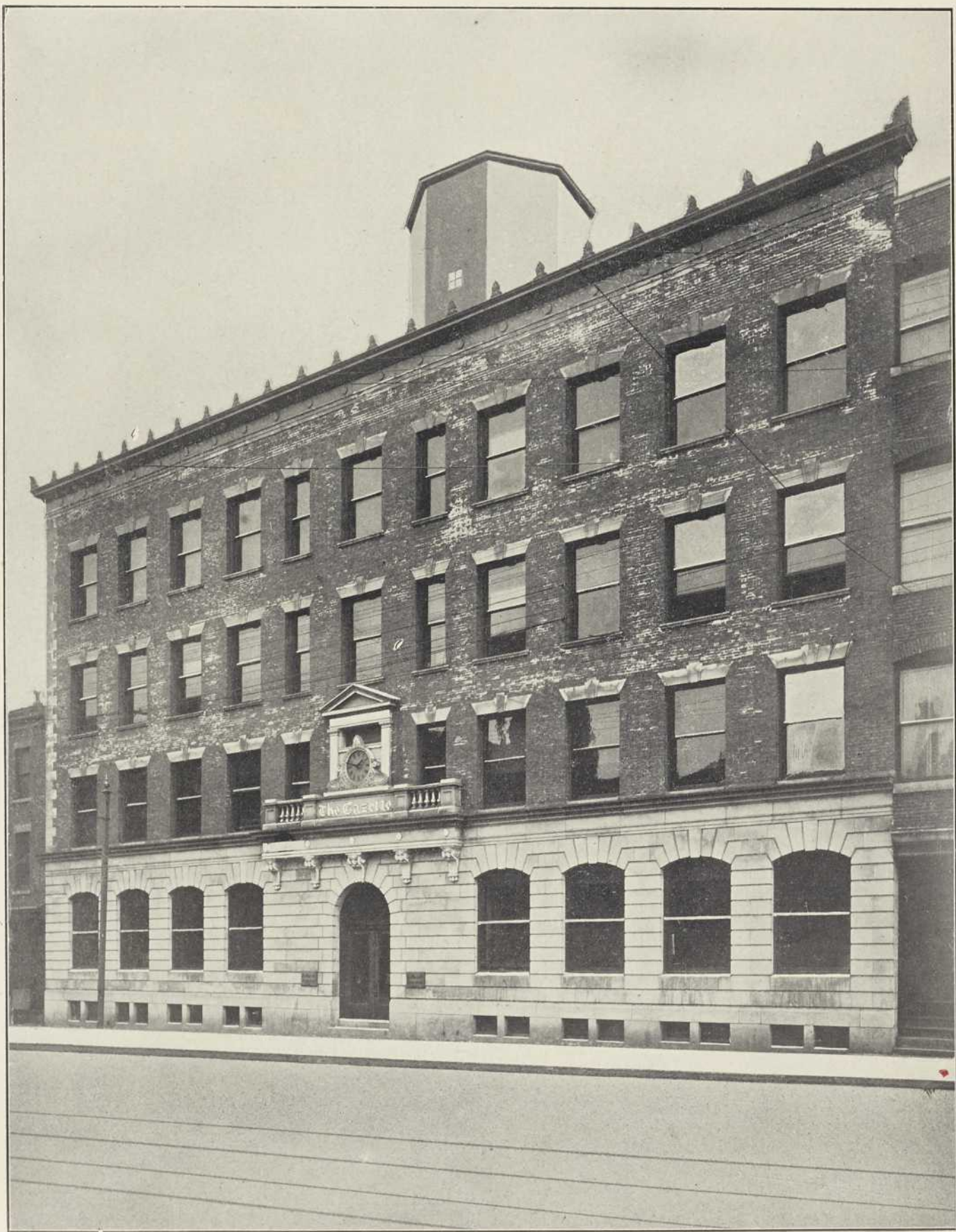
THE GAZETTE BUILDING
