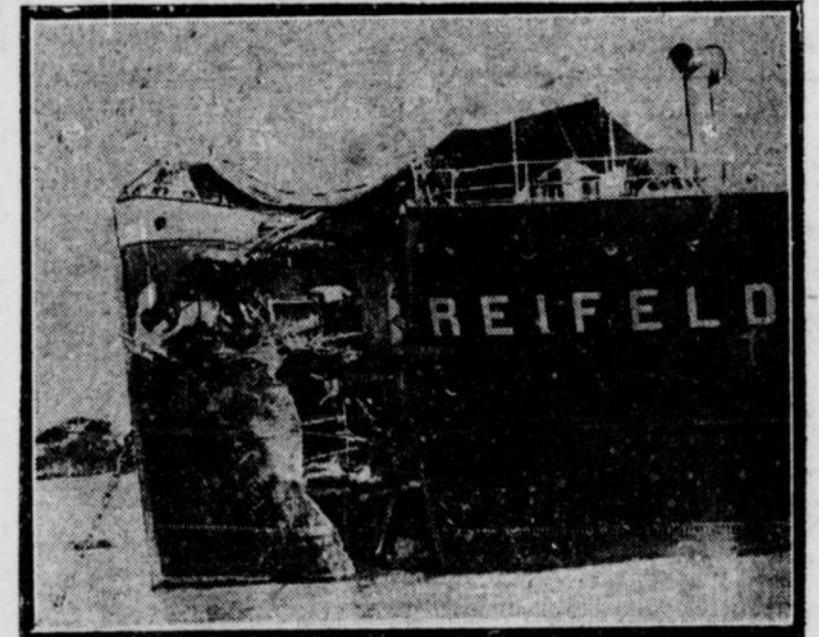
What the German boat Friefield looked like after being rammed by the American liner Katahdin. The watertight compartments saved the boat from sinking.
