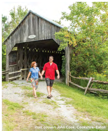
Pont couvert John Cook, Cookshire-Eaton
