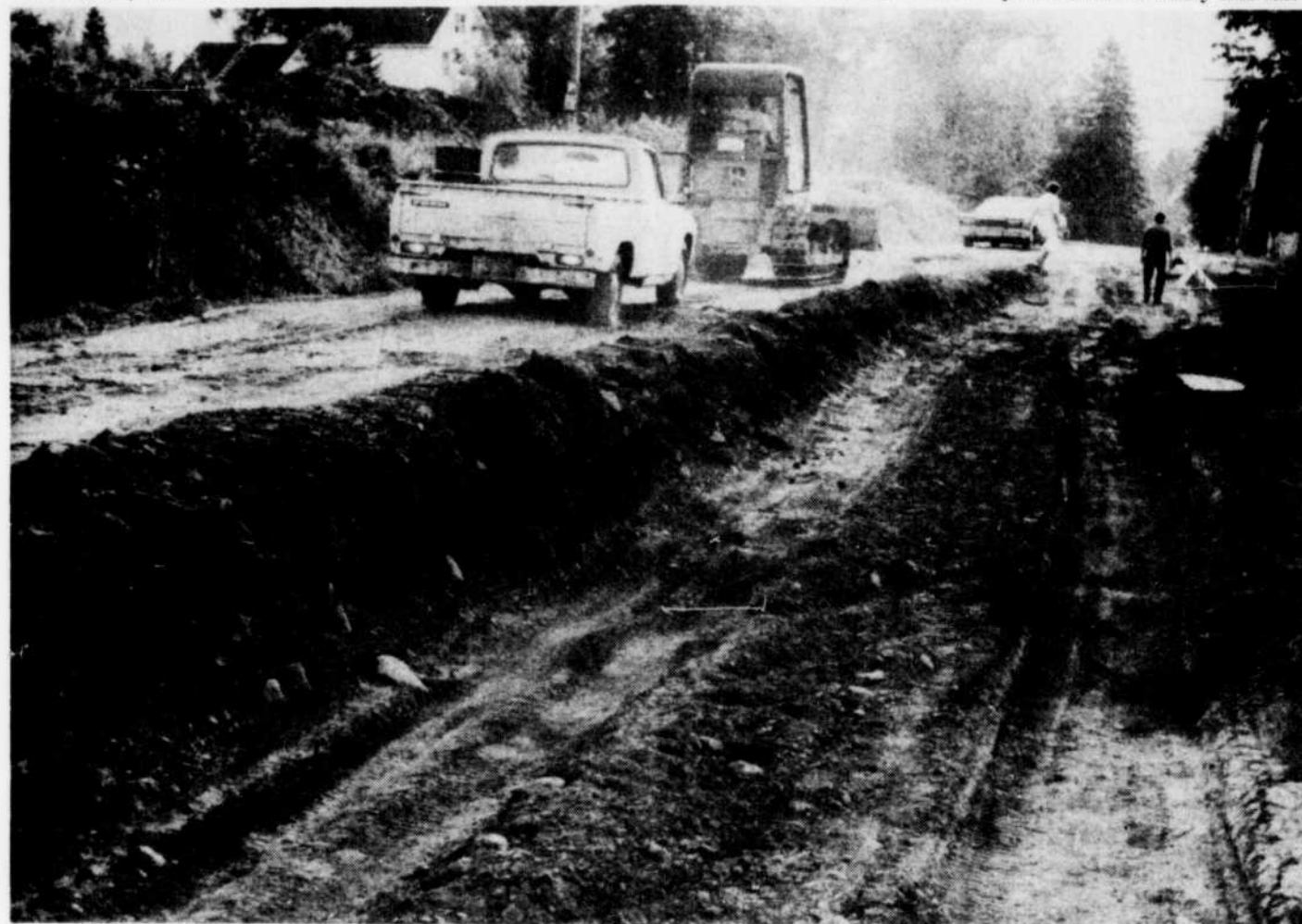
Just 'digging' it...
