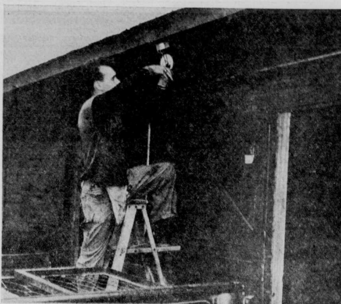
BROME FAIR PREPARATION — Jimmy Roderique of Cowansville is shown above installing light bulb fixtures in the horse stalls at the Brome Fairgrounds in preparation for the opening of the 99th Fair of the Brome County Agricultural Society which opens there Saturday and finishes on Tuesday. (Record Photo by Gerry Lemay)
