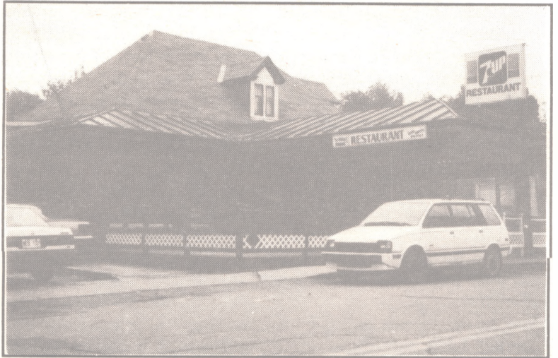
The Old Customs House at Rock Island has been turned into a restaurant called 'La Vieille Douane'. More pictures and story on Stanstead inside.
