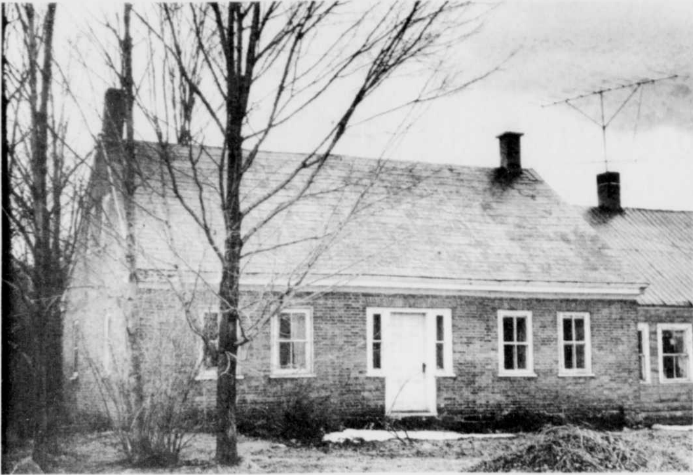
Bricks for this century home were made from clay taken along the Eaton River running just below the village.
