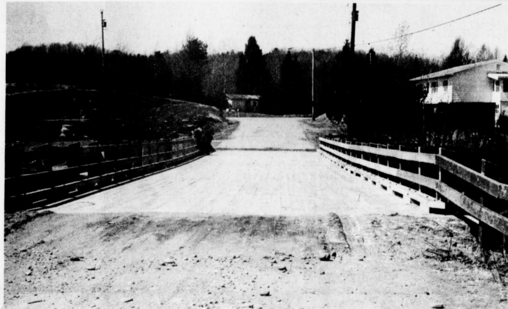
BRIDGE COMPLETED — The bridge over the Salmon River near Milby was completed late last week to replace the Bower bridge which was washed away three weeks ago. The residents, stranded on the other side, now have a link with the outside world. (Record photo: James Bruce)
