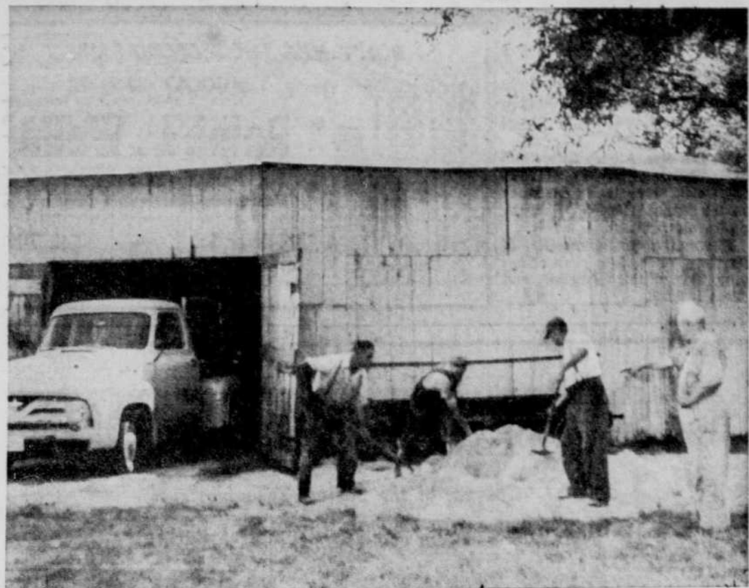
FAIR PREPARATIONS — Archie Sager, extreme right, superintendent of the Bedford Fair, supervises workmen preparing the Bedford Fair Grounds for the 127th annual Missisquoi County exhibition being held Aug. 20 to 22. The round building in the background, which has recently been converted into the Calf Club barn, formerly housed a covered merry-go-round in the first days of the fair over 100 years ago. (Photo by Gerty Lemay)
