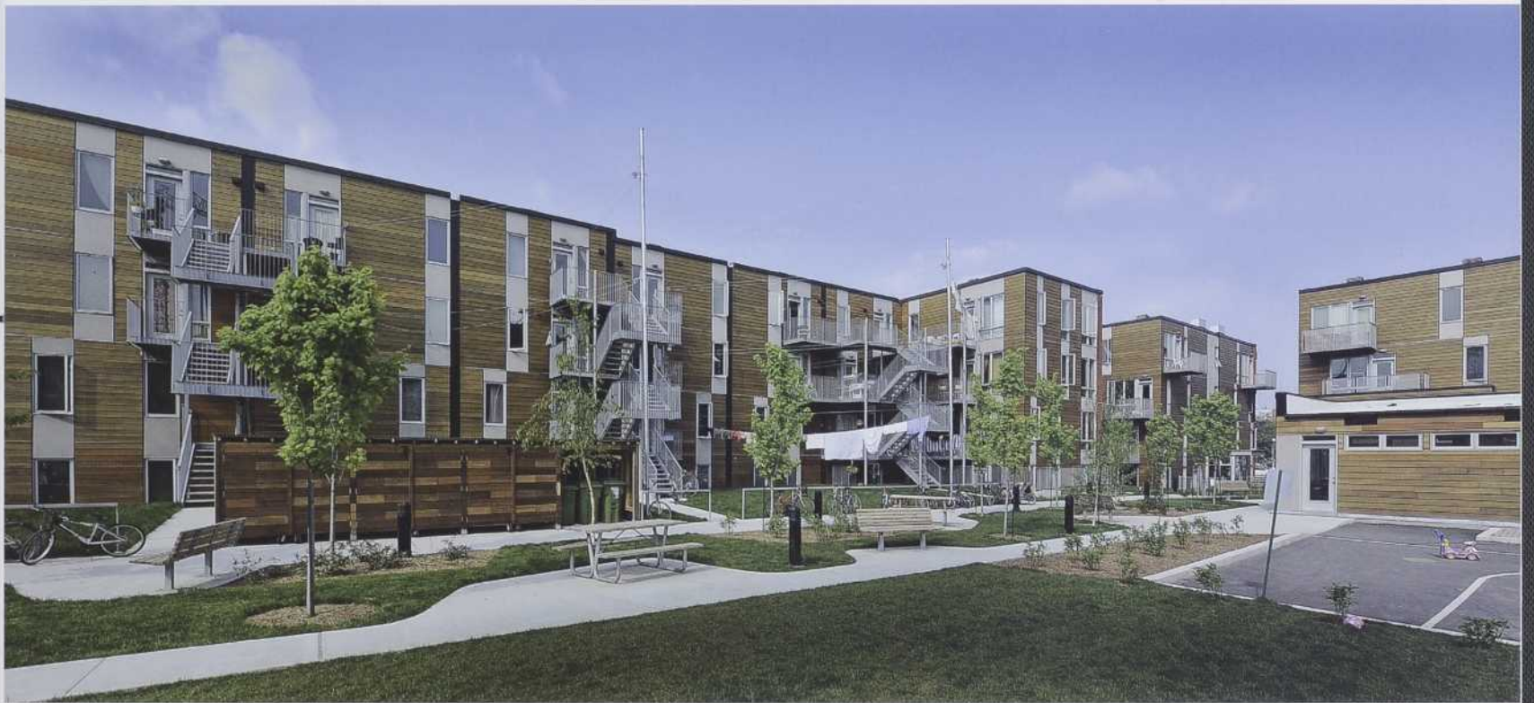
Photos: Nikkol Rot - The Holcim Foundation
