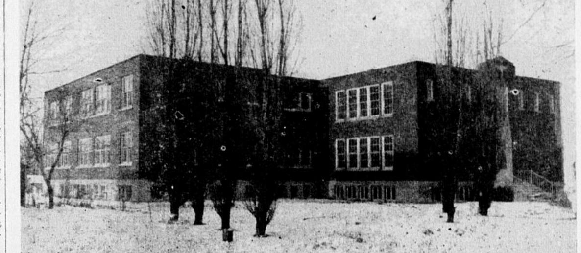
Shown above is the new addition that has been made to St. Joseph's School, Huntingdon, Que. The part showing the entrance at the right, is the original building. The part that is recessed and on the left is the new addition, so that building forms the shape of the letter L. A full story of this new school appears elsewhere in this edition. Not seen in the photograph, but at the left of the original building, is the Brothers' residence.
