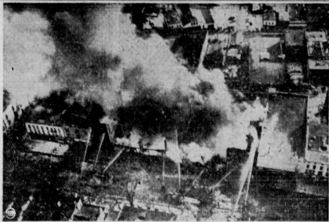
Up In Smoke — This aerial view shows part of the nearly three-million-dollar fire that killed one policeman and injured several firemen in Saratoga Springs, N.Y. The Red Cross declared it a disaster area as a whole city block was destroyed. The first started after an explosion in a bowling alley. (NEA)
