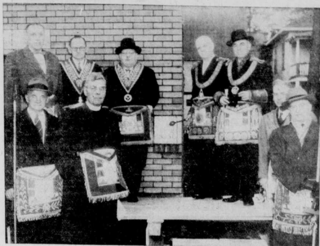
Cornerstone Ceremony — W. R. Bradford, Grand Master of Quebec, taps the ceremonial gavel on the cornerstone of the Ascot Masonic Lodge's new hall, under construction in Lennoxville, during Saturday's official dedication. Standing front row from left are Lawrence Parker, P.D.G.W.; Rev. Dr. Joseph Boucher, Past Grand Chaplain and R. Benton, of St. Lambert, past District Deputy Grand Master. Standing, rear, from left, are R. E. Mosher, acting Junior Grand Warden; C. Osborne, Senior Grand Warden; R. W. Louthood, Grand Secretary, Montreal; Mr. Bradford; J. W. McLean, Marshall, Deputy Grand Master of Quebec, and Geoffrey Lessard, Master of Ascot Lodge. (Record photo by Gerry Lemay)
