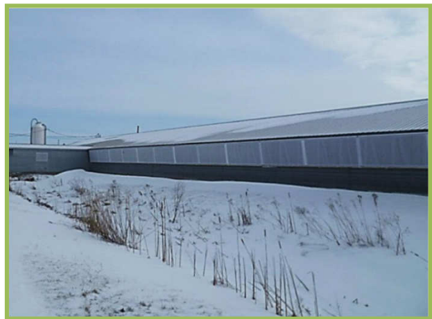
Figure 7 Buildings equipped with a curtain-type antimicrobial air filtration system
