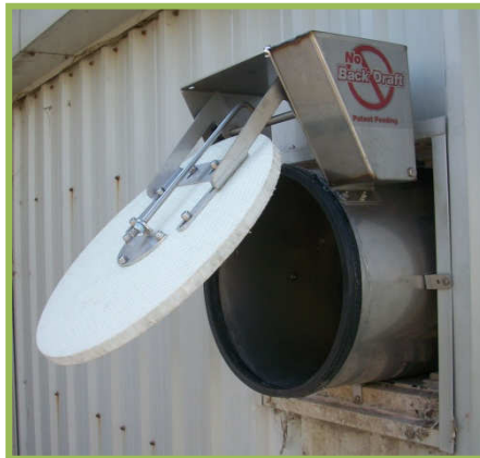
Figure 22 No BackDraft damper
