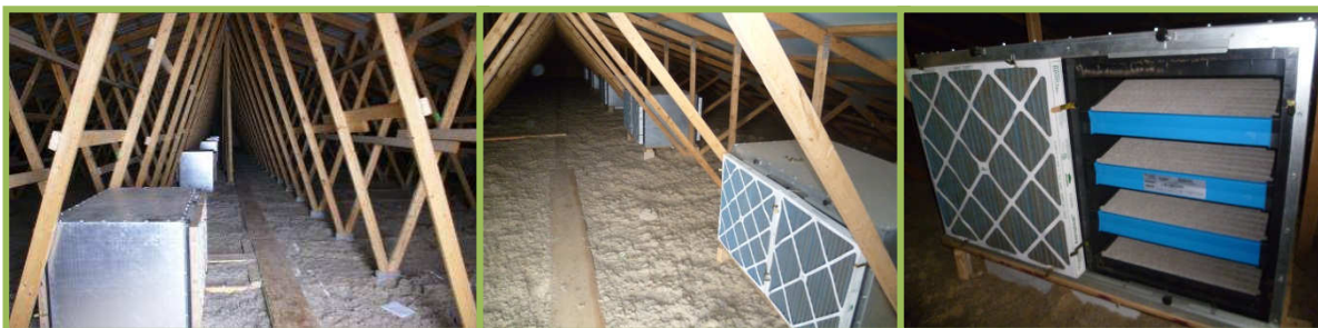
Figure 9 Filter boxes of mechanical filters installed on modular air inlets
