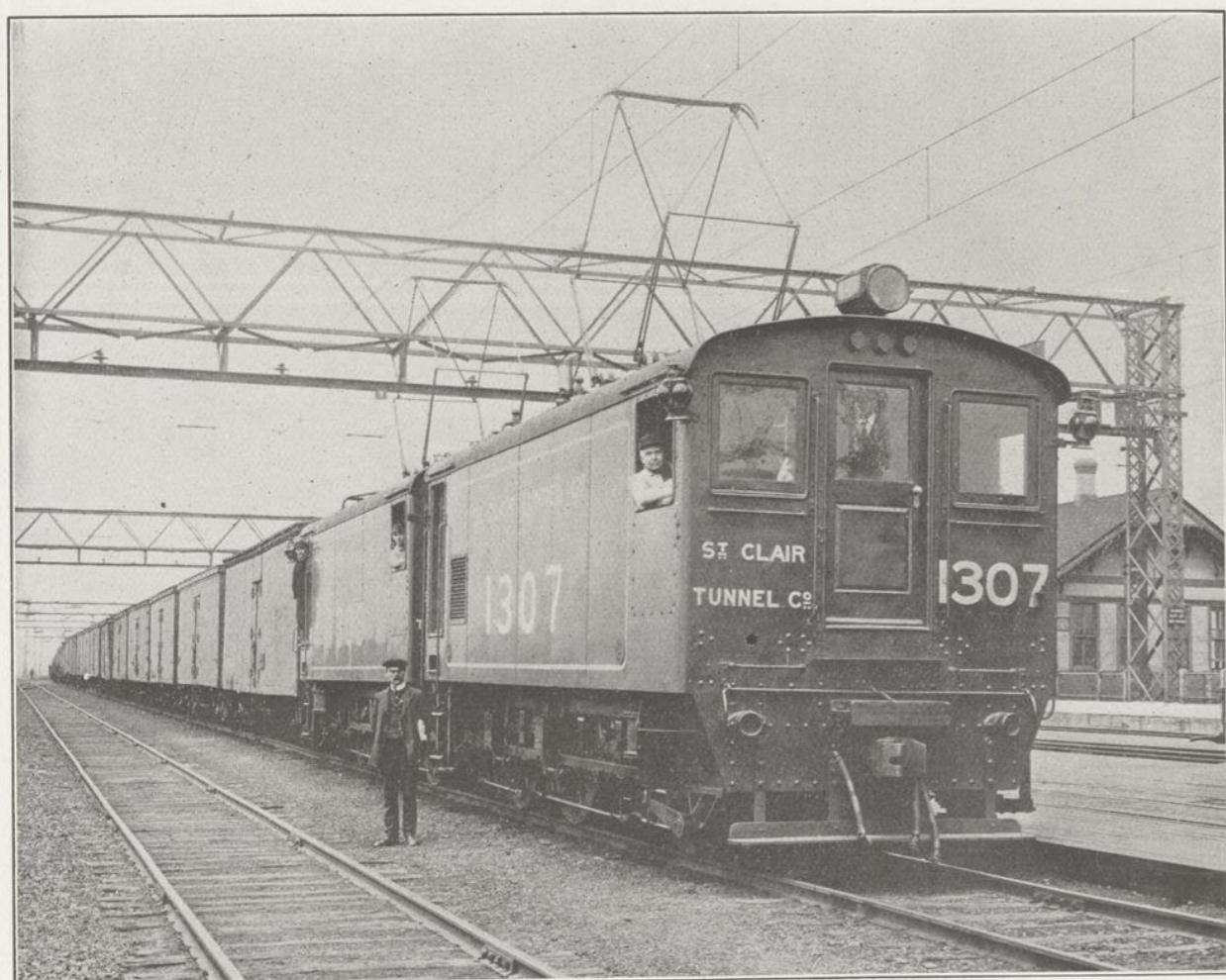
THE ELECTRIFICATION OF THE ST. CLAIR TUNNEL —One of the powerful electric locomotives that now hauls Grand Trunk trains through the tunnel beneath the St. Clair River, connecting Canada with the United States. These locomotives have taken the place of the mighty steam moguls which used to do this work.
