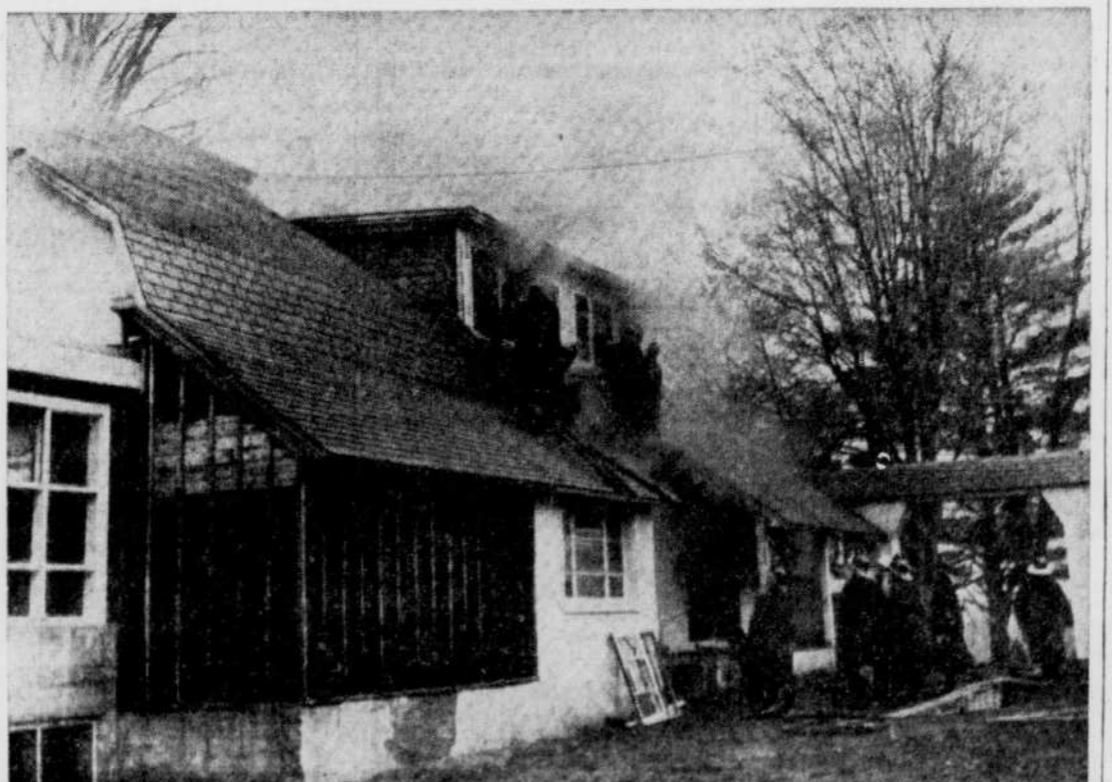
Cowansville Fire — Damage estimated at $4,000 was caused by fire which broke out in "The Cowansville Garden," early Monday morning. The property, formerly owned by Albert Gillies, a metal worker, was recently purchased by Judge Mason Lorange of Montreal as a home for retired people but was unoccupied at the time of the blaze. (Record photo by F. Gillespie)
