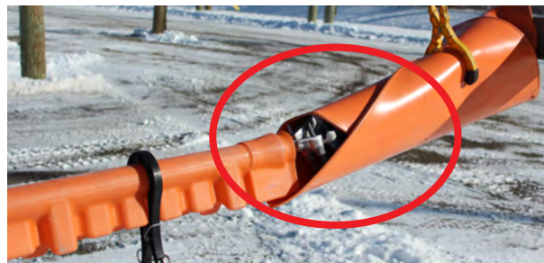
Incorrectly superposed conductor covers
