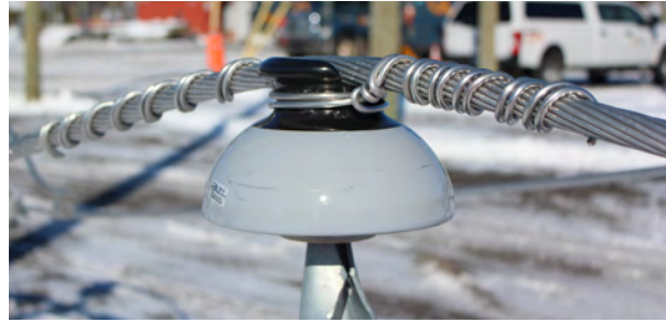
Tie wires in good condition
