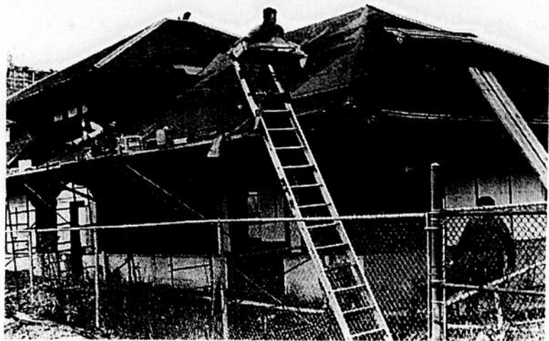
Repairs are made to the roof of the controversial CP train station in November to prevent its further deterioration.
