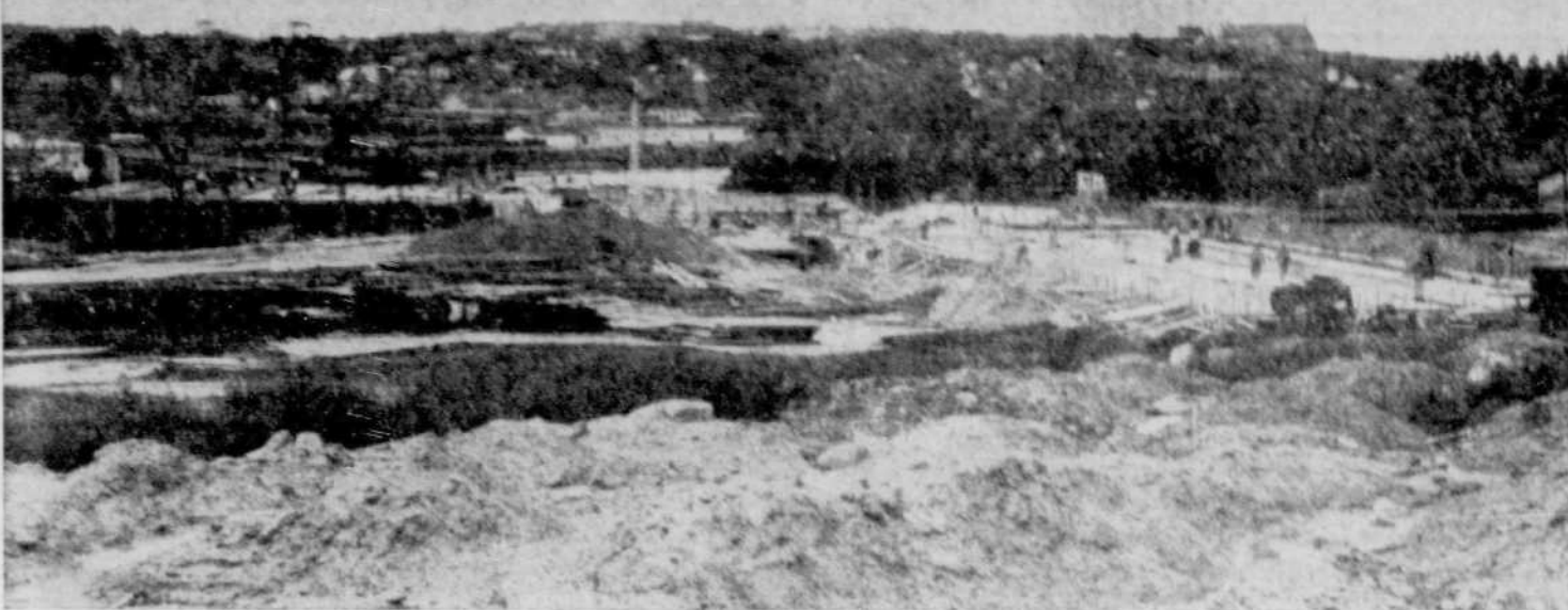
NEW SCHOOL --- Construction work is progressing rapidly for the new Superior School being erected by the Sherbrooke Roman Catholic School Board. The new structure, at the corner of Galt street east and Bowen Avenue south, will replace the school now located on King street. The present Superior School will become a normal school for girls. (Record photo by Gerry Lemoy).
