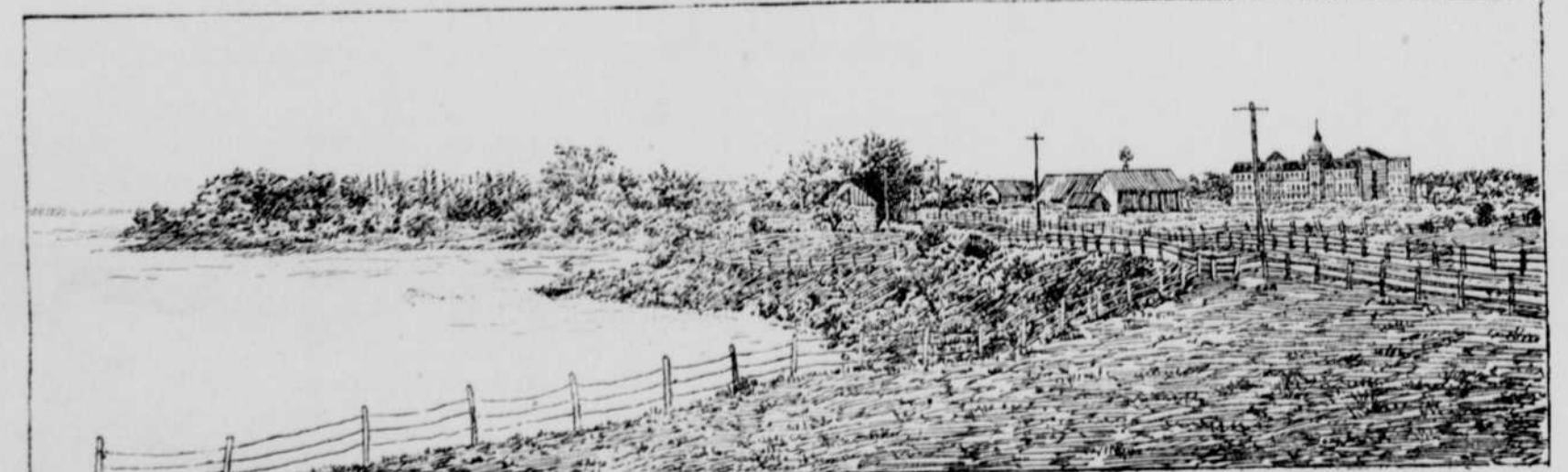
VIEW OF HOSPITAL FROM FOOT LACHINE RAPIDS.
