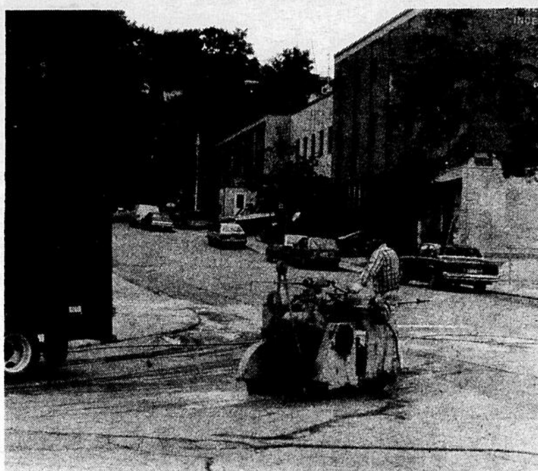
A workman makes the first road cut Monday morning at the corner of Stanton street as the reconstruction of Côte St Antoine road begins.
