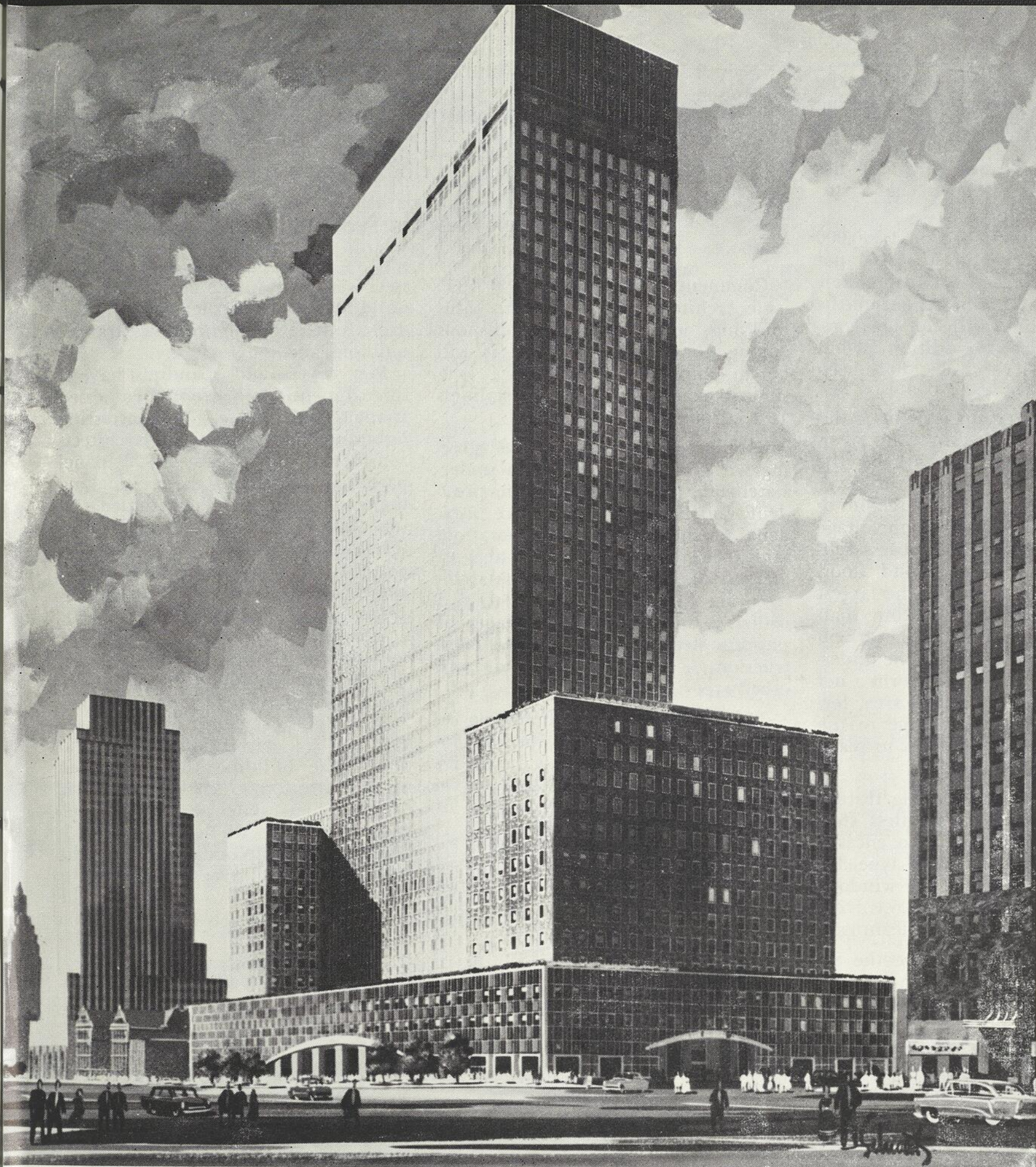
The walls of this skyscraper have been encased in some 7,000 panels of stainless steel sheet. All windows are framed in stainless steel, revolving from the inside for ease of cleaning. This 42 story building was erected in the Grand Central Station area, in New York.
