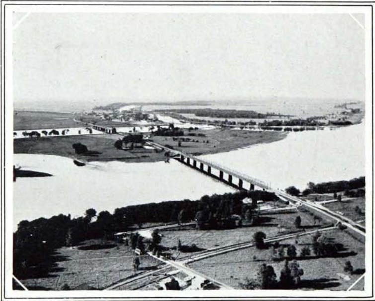
Charlemagne Bridge, on Highway No. 2
