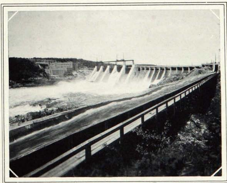
Dam and power-house on a Quebec river
