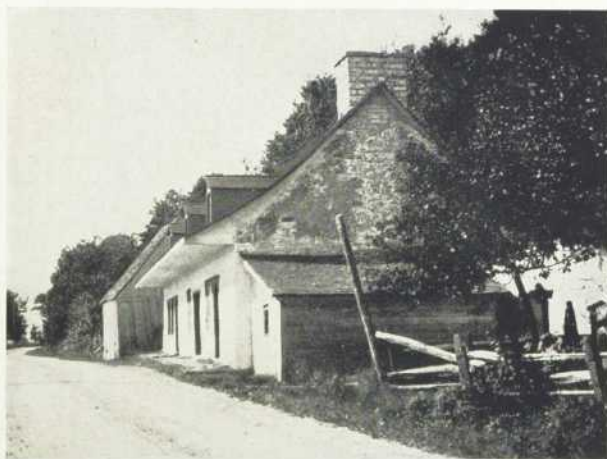
Fig. 3. On the road between Montmorency and Beauport. The Quebec Type.
