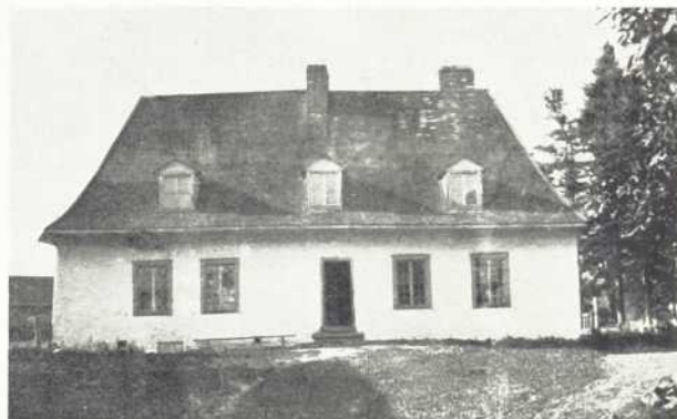
Fig. 4. On the road between Montmorency and Beauport. The hipped roof type.
