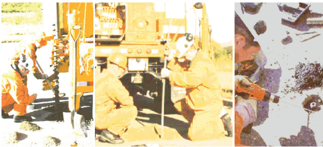
Installing a frost probe in the pavement
