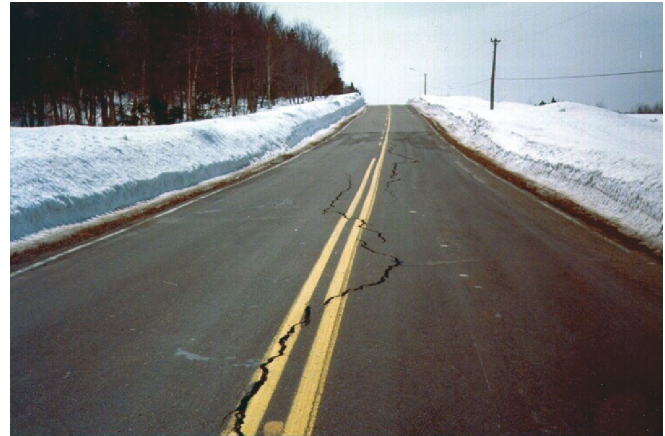
Longitudinal cracking, as depicted in Figure 2
