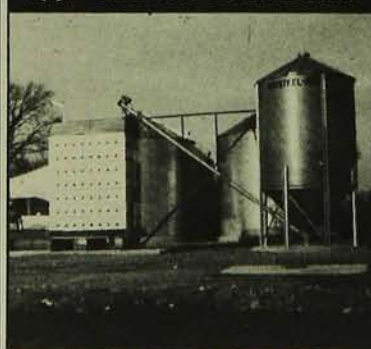
FERME Mc GERRIGLE, ORMSTOWN
