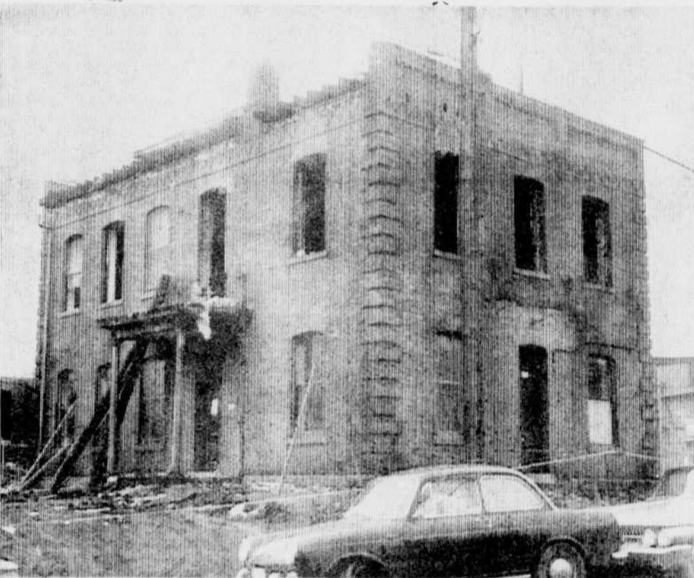
TO MAKE ROOM FOR PARKING LOT — The old Registry Office on Bank Street is being demolished to make room for another parking lot. The office moved recently to its new quarters on Palace Street across from the Court House. The old building is an historic site. The first Anglican church in Sherbrooke was established on that spot. (Record photo by Gerry Lemay)
