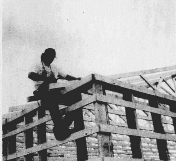
Morgan Arthur nailing the last rafter.
