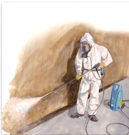
Figure 3: Washing technique with low-pressure water jets
