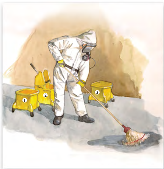
Figure 2: Wet clean-up technique with three pails
