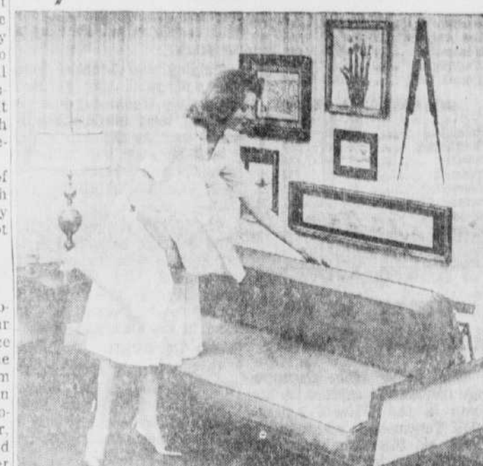
A TRANSFORMATION — A quick bed in this modern room is a sleek sofa by day. Latex cushion is made up with sheets and blankets concealed by upholstery covering. Rolling back section forward readies bed for the night. Pillow is housed in compartment in back.
