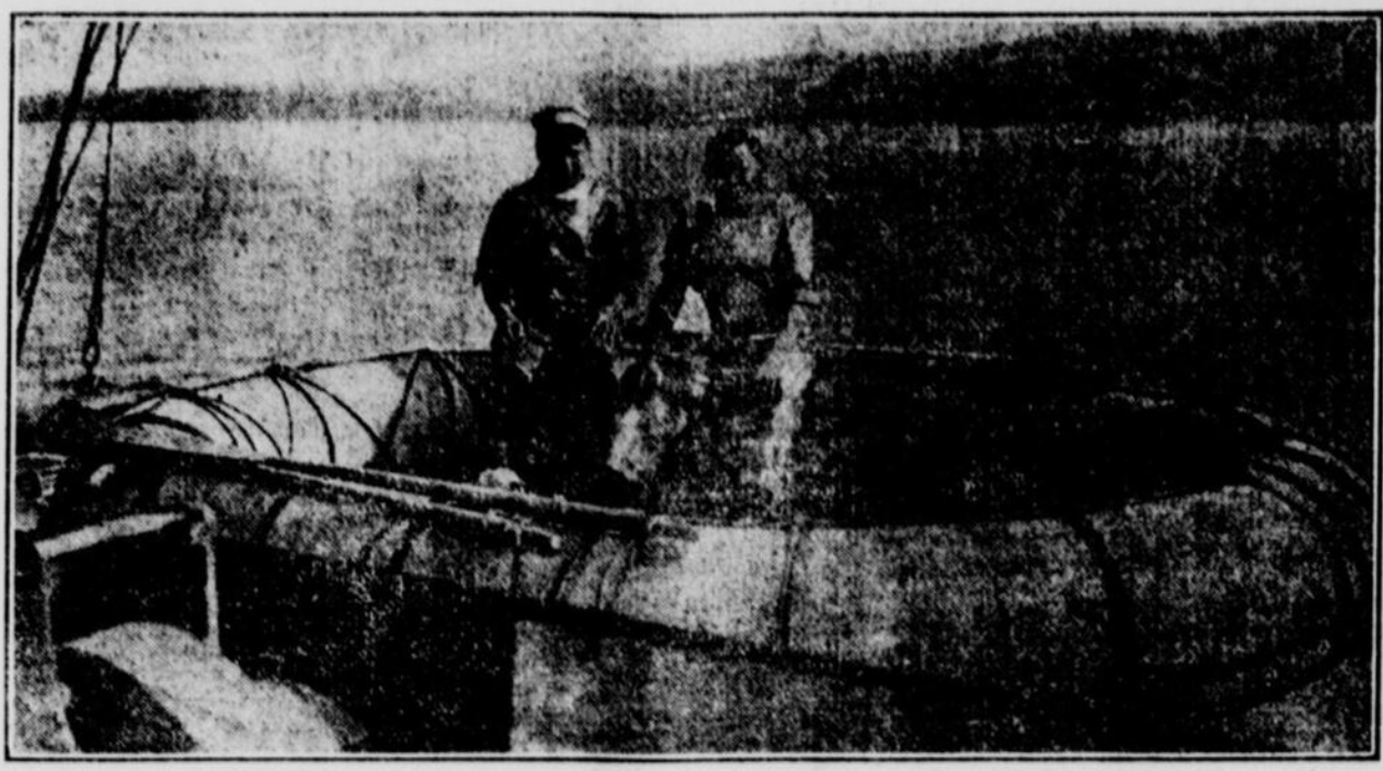
The life-buoy lifeboat, which has now been adopted for use by main ships of the British Navy. These buoys can sustain thirty men on the inside; the photograph gives a good idea of the size of the buoy in comparison with the men sitting in it.
