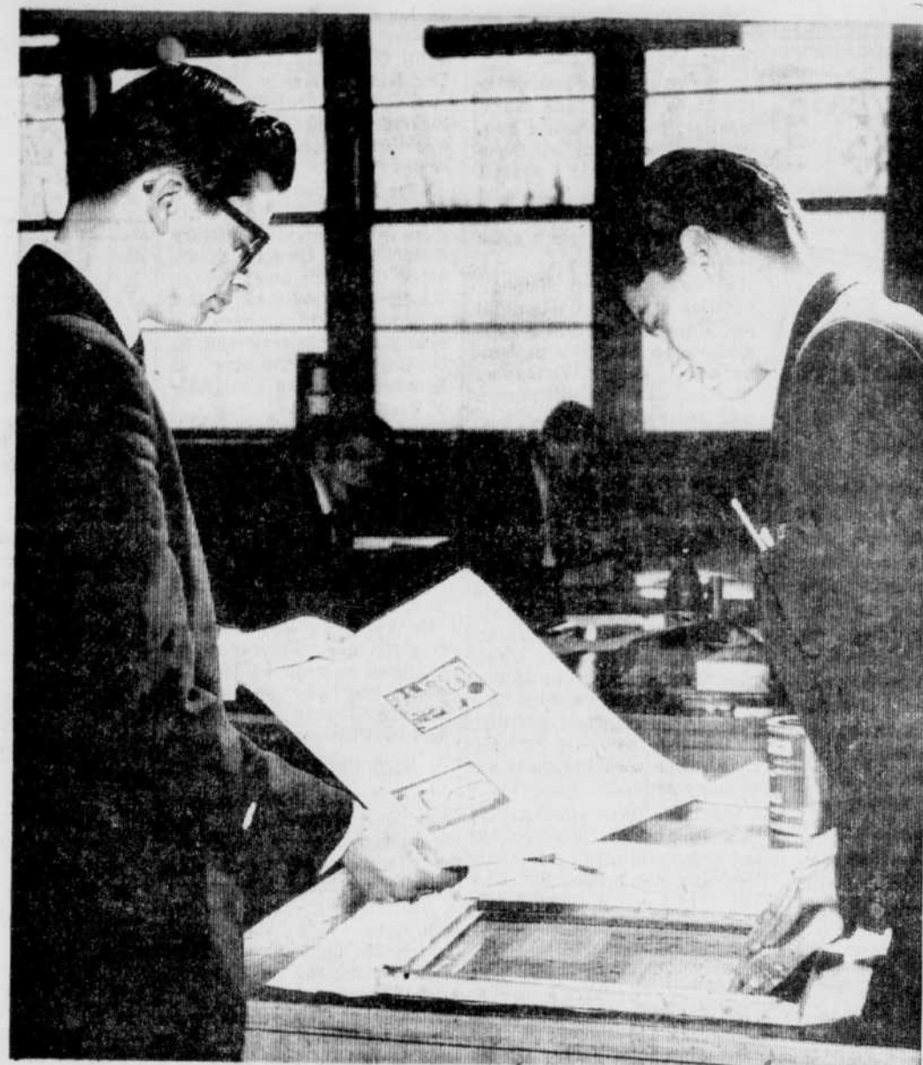
SILK SCREEN PRINTING — A form of reproduction of art work. Shown is a frame with open areas to allow the color to be pressed through with a squee-gee.
