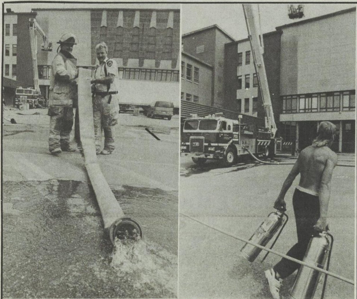
On a hot tar roof A fire which erupted while roofers were putting a new top on the Séminaire Salésien was put out quickly by construction workers armed with extinguishers. The fire department, which arrived within minutes, gave a final dousing to embers and ensured all flames were extinguished. The fire caused little damage and the roofers went back to work after cleaning up the water.
