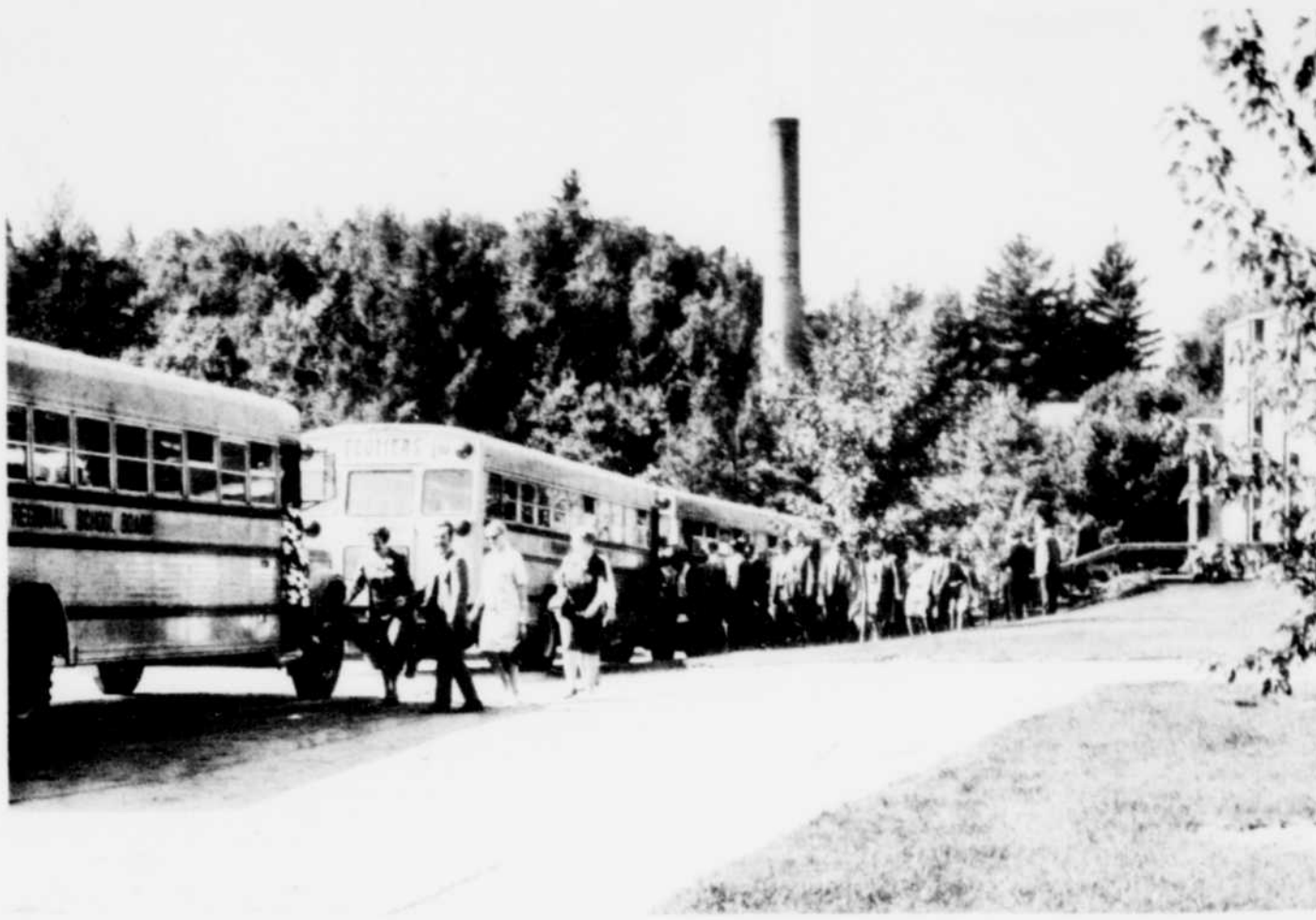
SCHOOL VISIT — Alexander Galt Regional School teachers visited the construction site of their future school on Tuesday. Seen above teachers are mounting buses at Bishop's University
