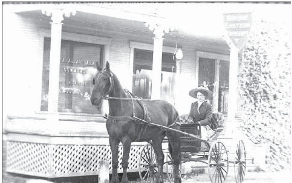
Eastern Townships Bank office, possibly in Leeds, shortly after its acquisition by the CIBC, ca. 1912. Both bank names are visible on the window. (P020 E.T. Heritage Foundation fonds)
