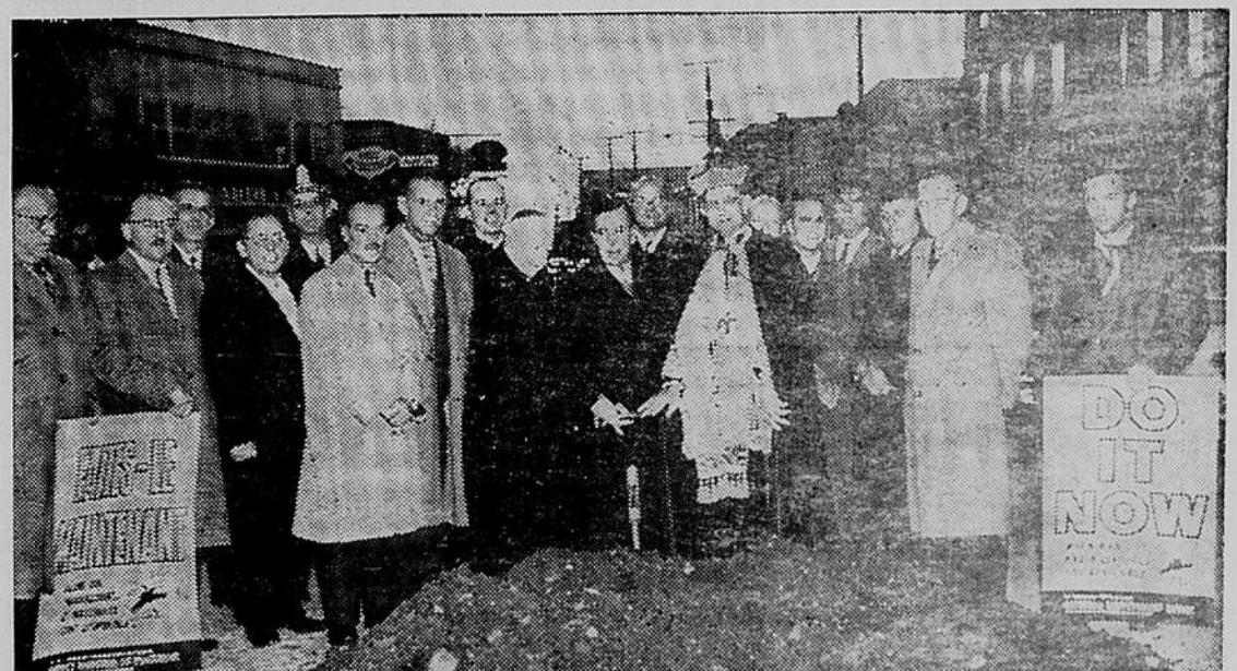
Their Excellencies Bishop Langlois and Bishop Caron blessed the start of Valleyfield's Winter Work Program last Monday afternoon when excavation work was started on the extension of the Valleyfield City Hall. Mayor Robert Cauchon moved the first shovel of earth. Others in the picture are aldermen, city officials and Messrs. Laurent Boyer and Lalonde, extreme left and right, of the Employment Office. Missing at the ceremony were representatives of the Federal and Provincial Govern... the two sources who are providing 90 per cent of the labor for the Winter Works Program. (Photo - Peter Rozon)
