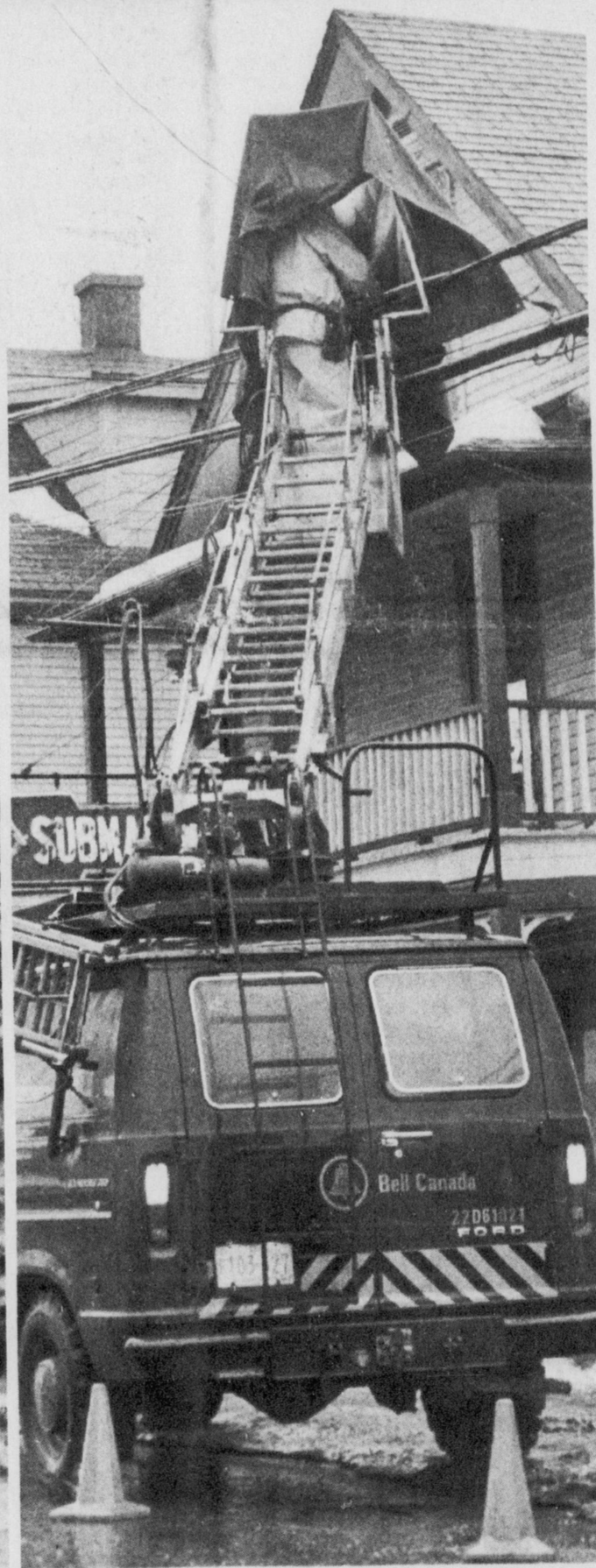
Right, a Bell maintenance man works in reasonably dry surroundings.
